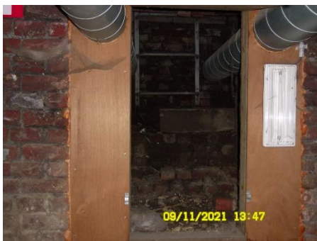
Escape route with ladder (basement -2)
