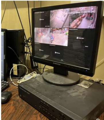
Server room monitor
